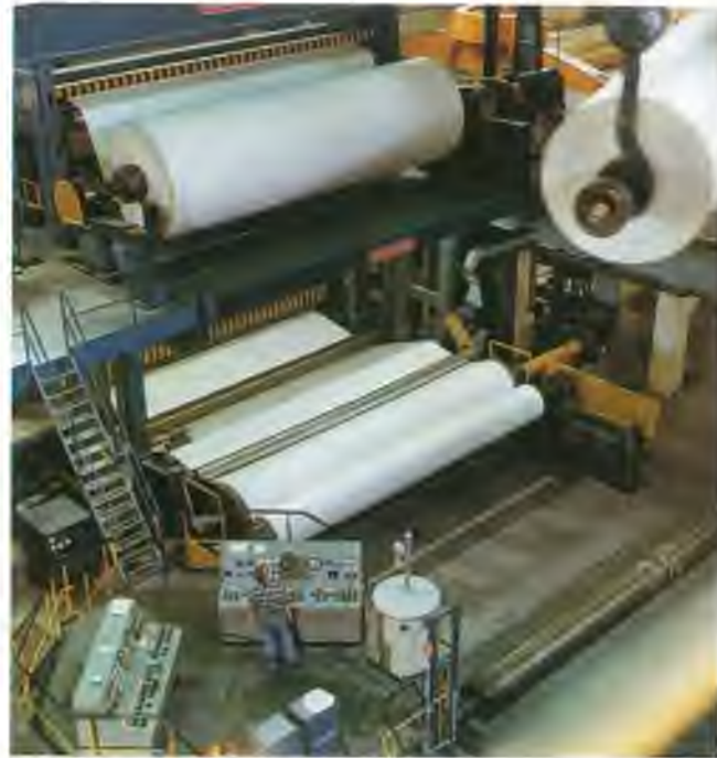
Machinery in a paper mill. Drives and controls are designed to the strict quality requirements of calender systems with web widths of
