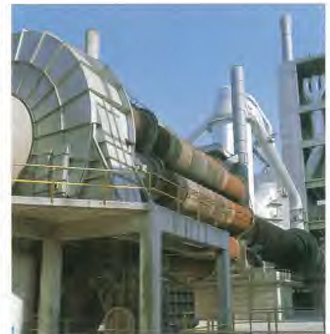
Rotary kiln plant capable of producing 3,000 tons of cement per day. Siemens provides the cement industry with electrical engineering equipment such as power supplies, drives, and automation systems.
