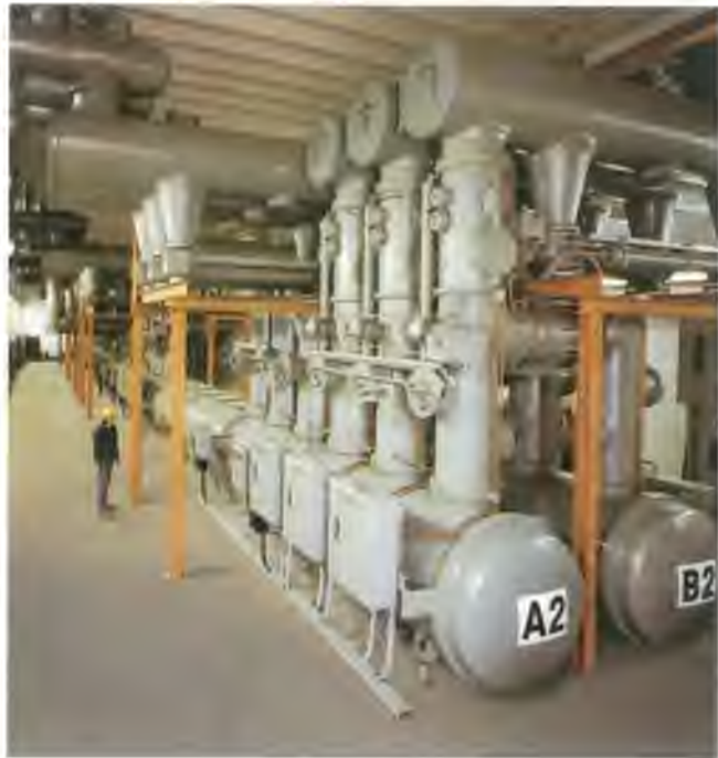
Metal-enclosed medium- and high-voltage power breakers using sulfur hexafluoride (SF 6 ) as the insulating gas are available for voltages ranging from 6 kV to 800 kV.
